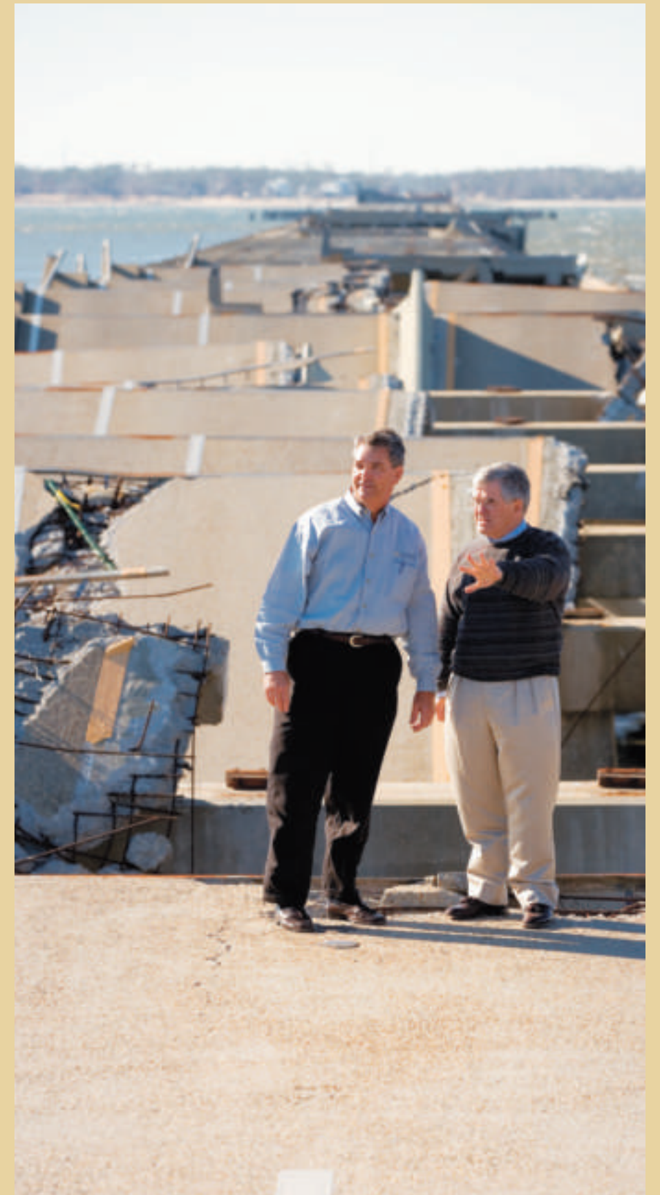
Atlanta Fed New Orleans Branch Director Dave Dennis (left) shows Federal Reserve Board Governor Mark Olson the destroyed bridge over Bay St. Louis in Mississippi. Dennis talked about the plans already in place for rebuilding the Mississippi coast.
